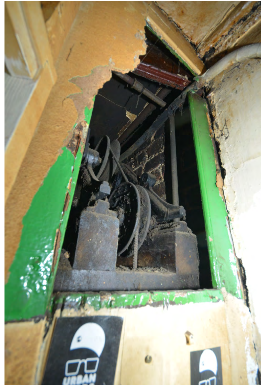
Plate 120: Detail of dumb waiter mechanism
