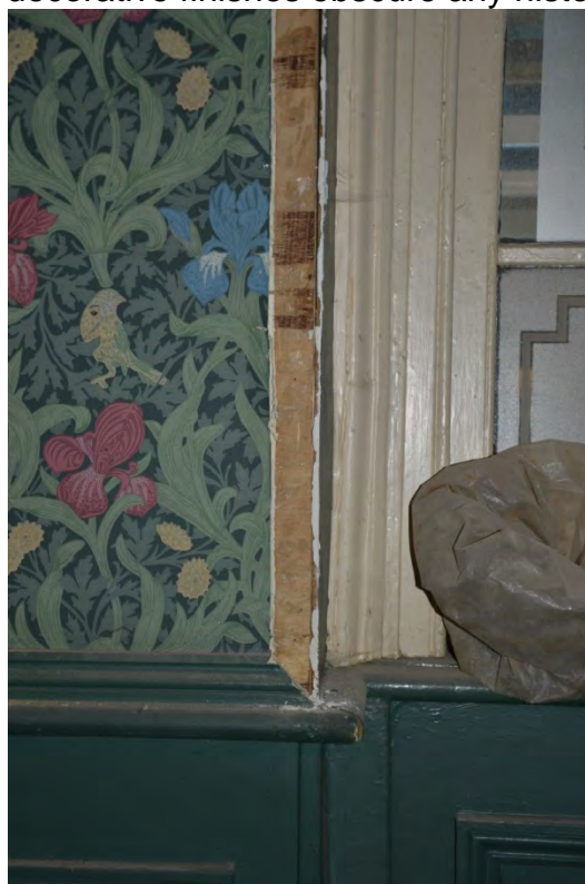
Plate 19: Modern plywood revealed during recent works
