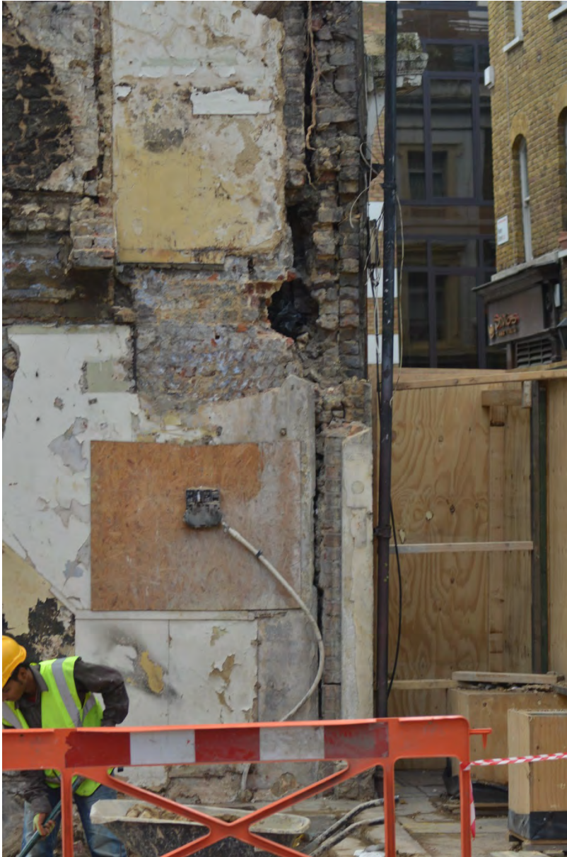
Plate 53: Detail of structural crack, west end of north elevation
