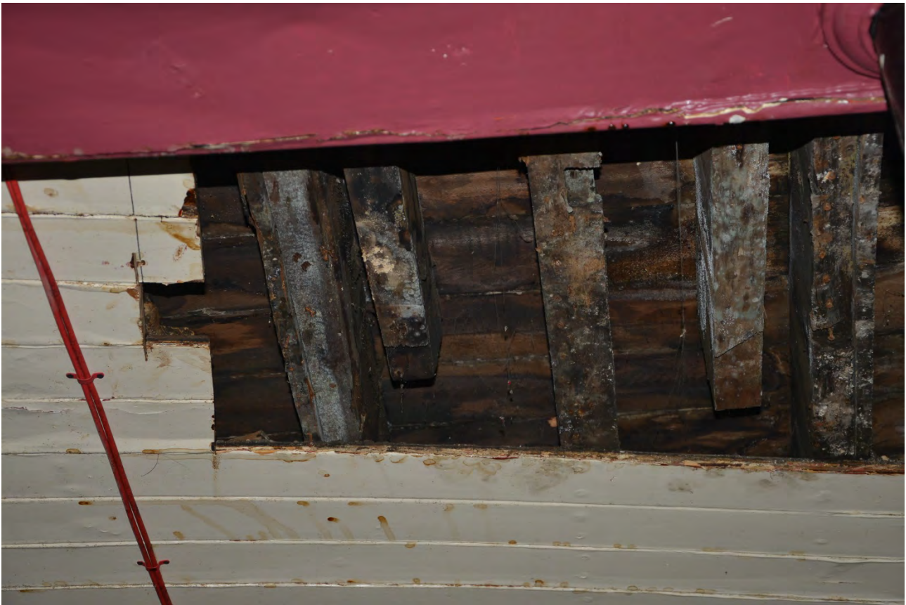
Plate 174: Exposed ceiling / first floor timbers, area A
