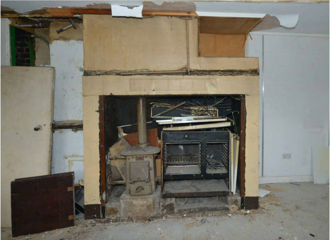
Plate 123: Fireplace exposed as part of alteration works
