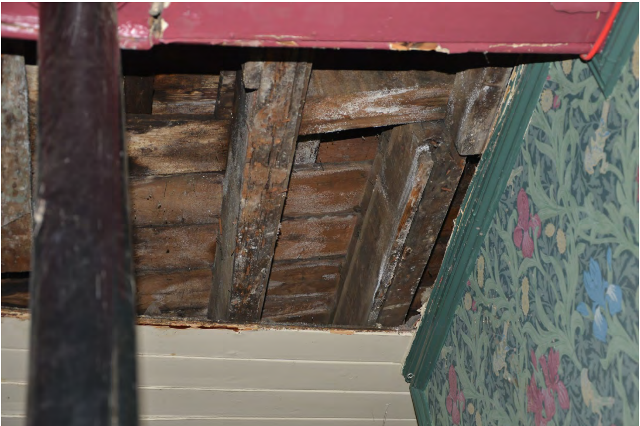
Plate 175: Exposed ceiling / first floor timbers, area A
