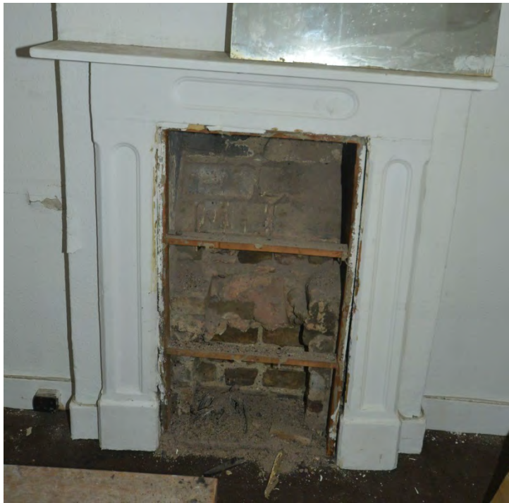
Plate 136: Detail of unblocked fireplace
