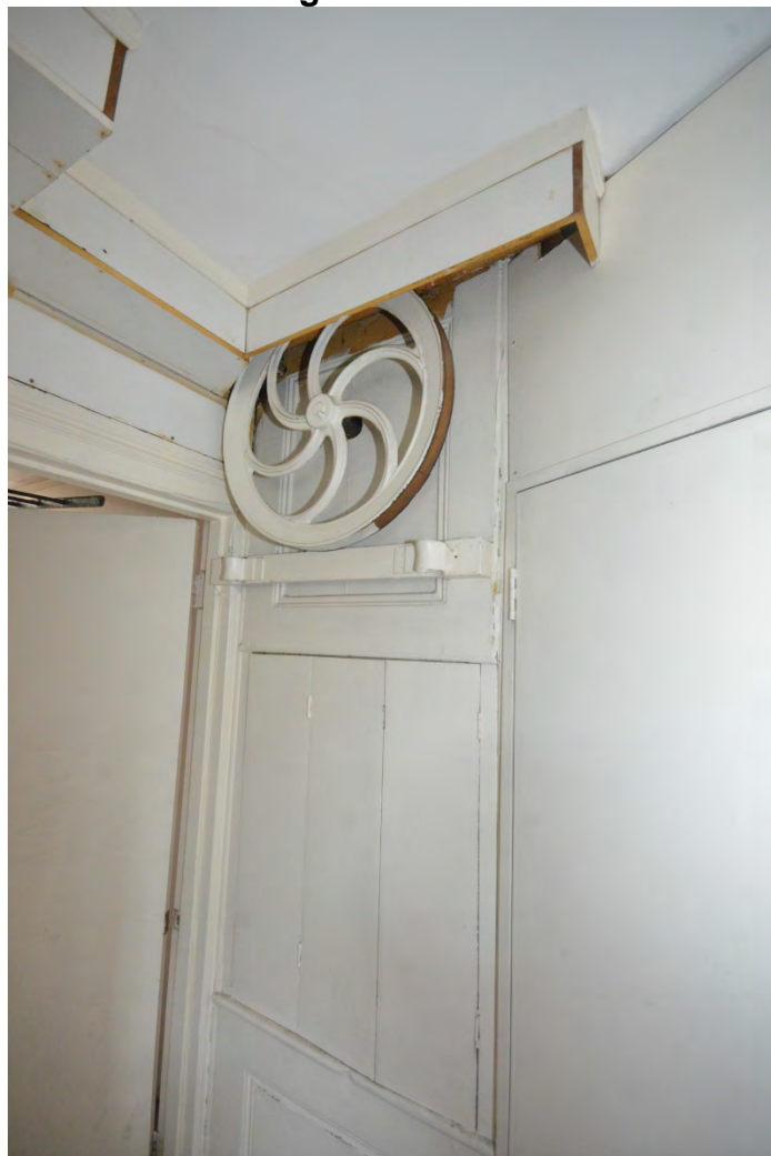
Plate 122: Pulley wheel and hatch, dumb waiter
