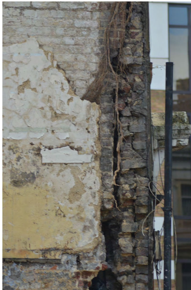
Plate 52: Detail of structural crack, west end of north elevation
