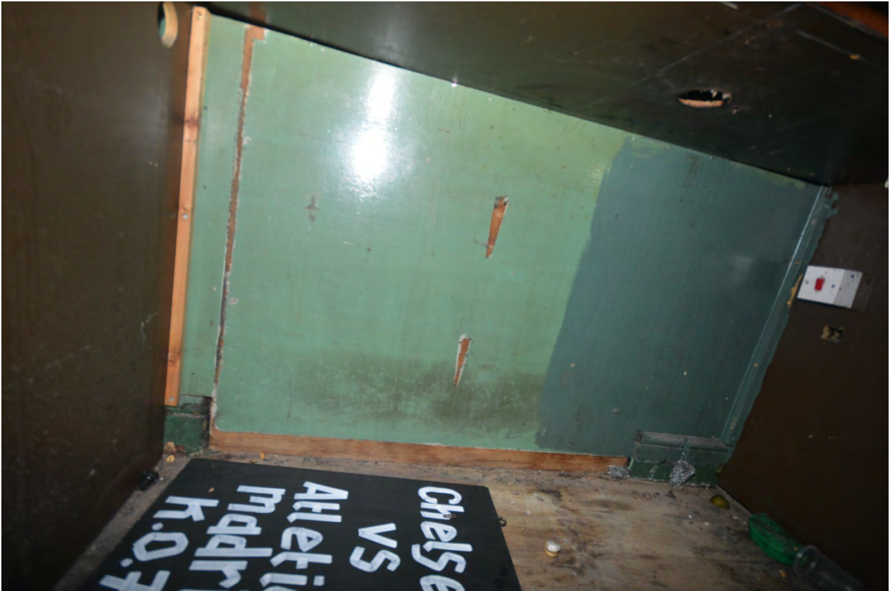
Plate 168: Former refrigerator recess showing board blocking fireplace
