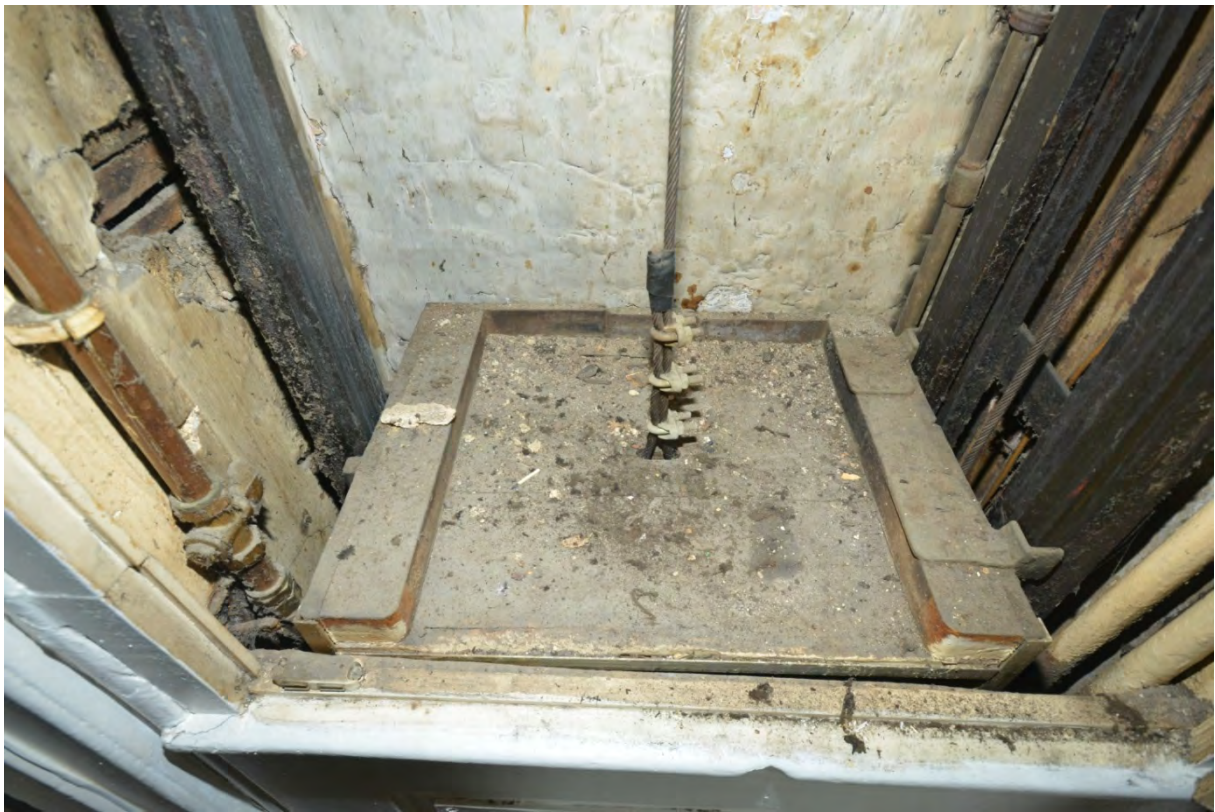
Plate 121: Top of dumb waiter 'carriage' viewed from access doors
