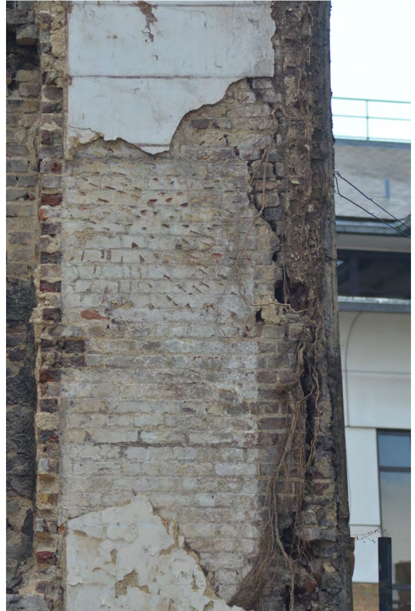
Plate 54: Detail of structural crack, west end of north elevation
