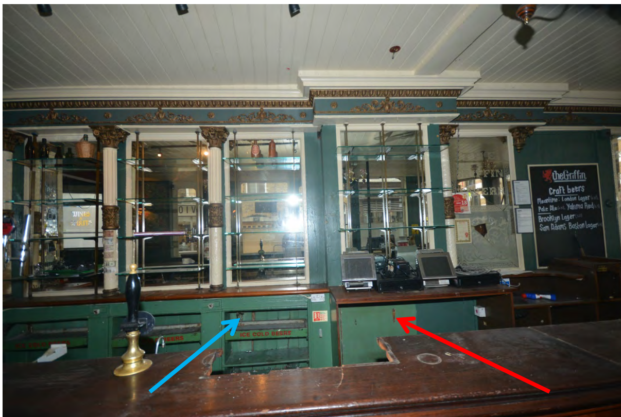
Plate 171: Location of fireplace (arrowed red) and wallpaper (arrowed blue) The above photograph clearly shows the chimneybreast leading up from the fireplace.
