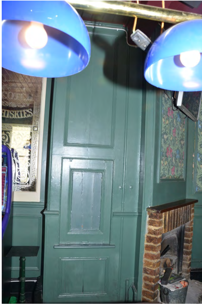
Plate 20: Panelled enclosure for the dumb waiter
