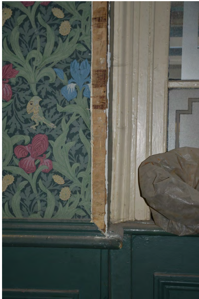
Plate 173: Plywood boxing in of soil pipe
