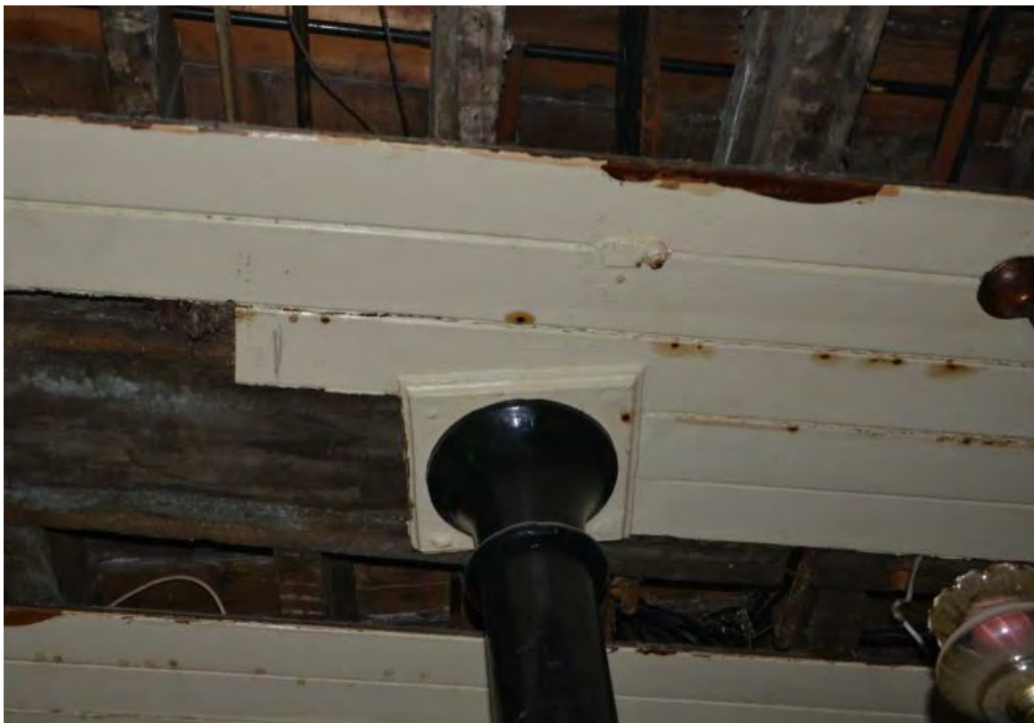
Plate 3: Lath & plaster marks revealed beneath tongue and groove
